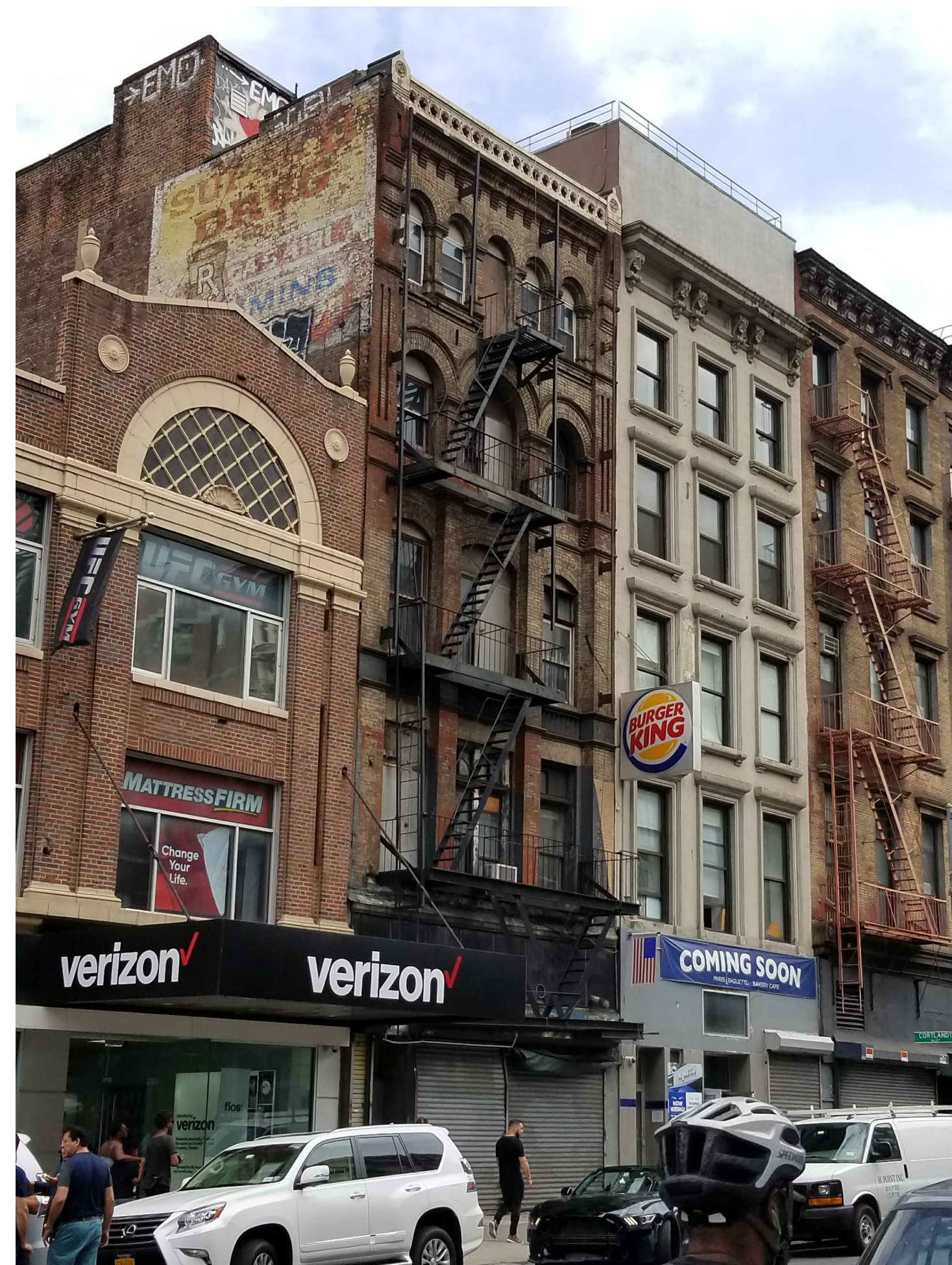
01 OVERALL EXISTING BUILDING VIEW
