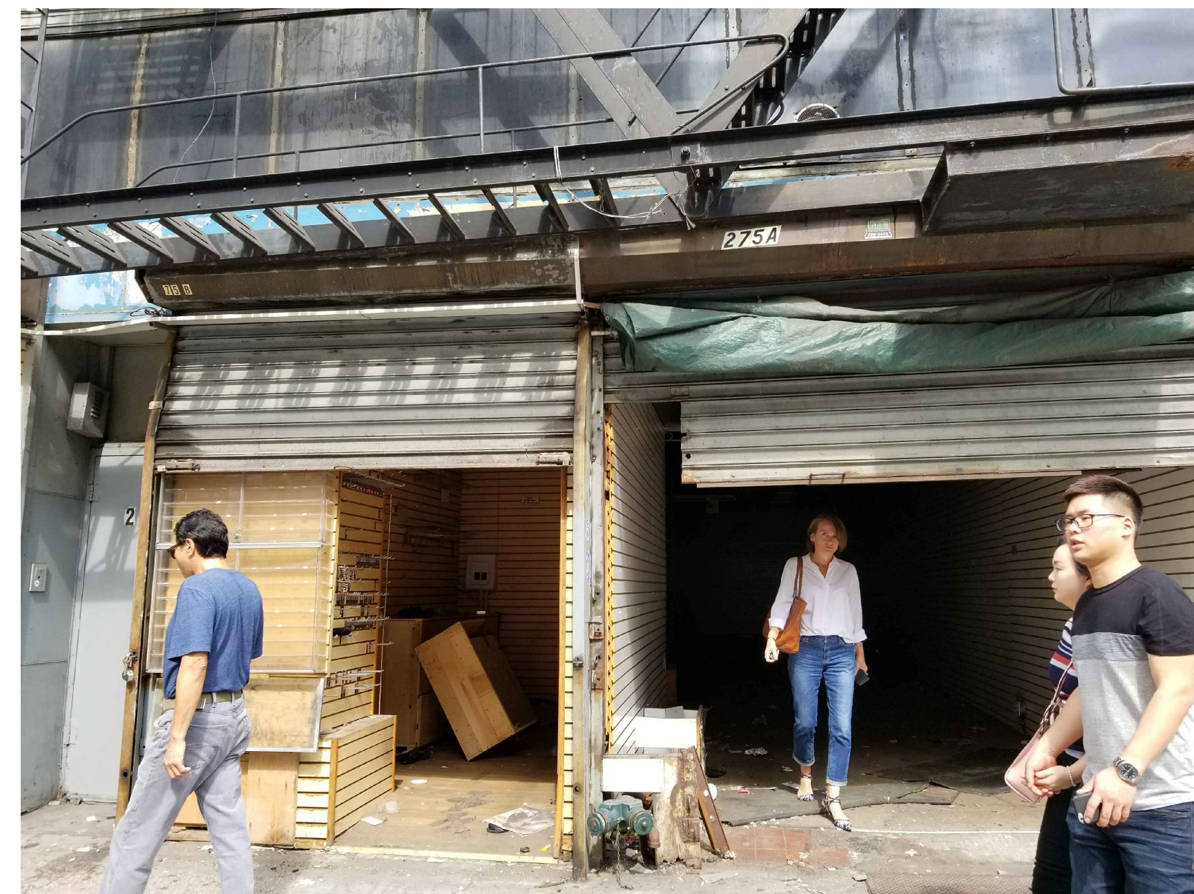
05 EXISTING ROLL DOWN GATES AND RETAIL VIEW (OPEN)
