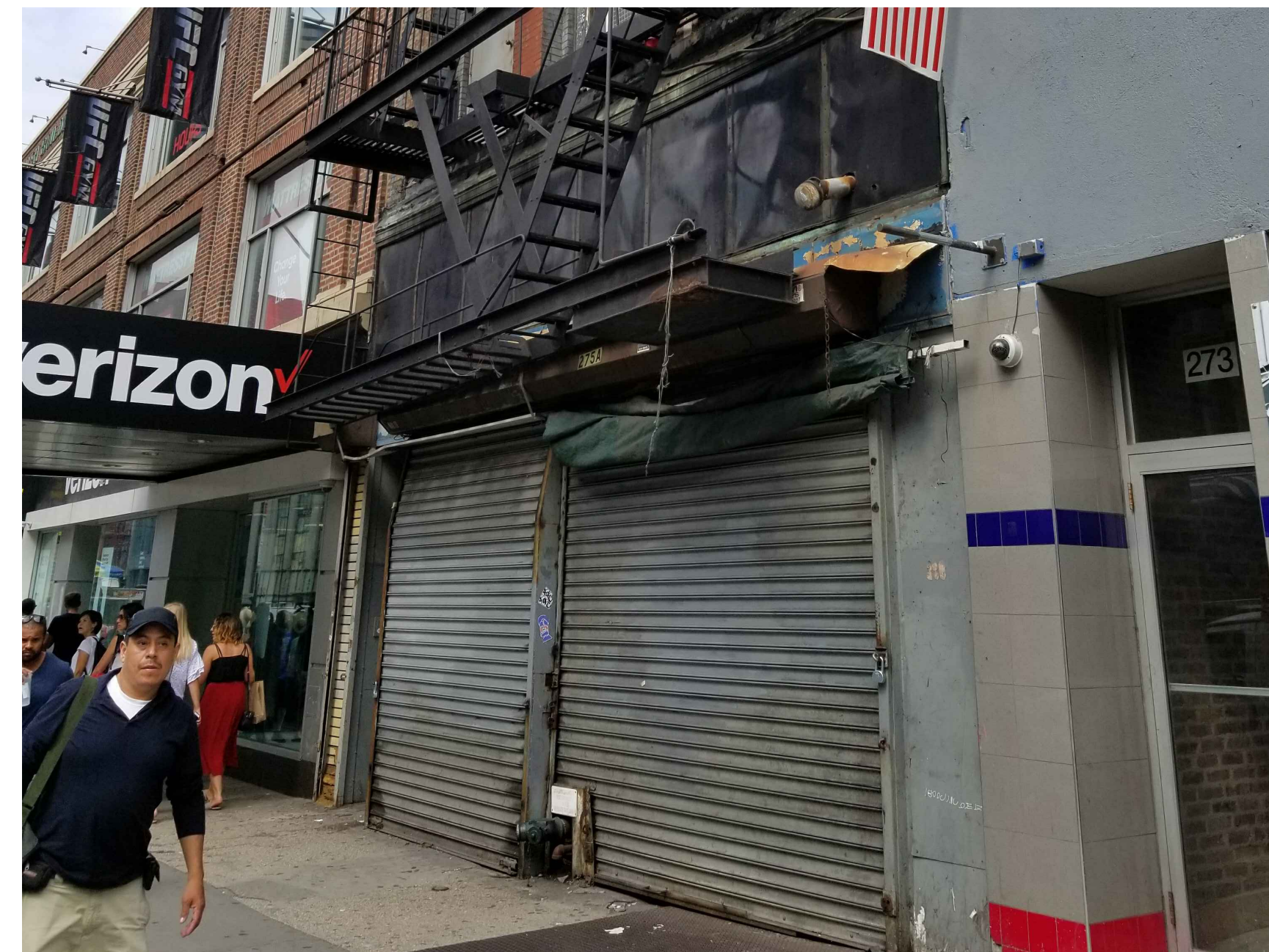
04 EXISTING ROLL DOWN GATES AND RETAIL VIEW (CLOSED)
