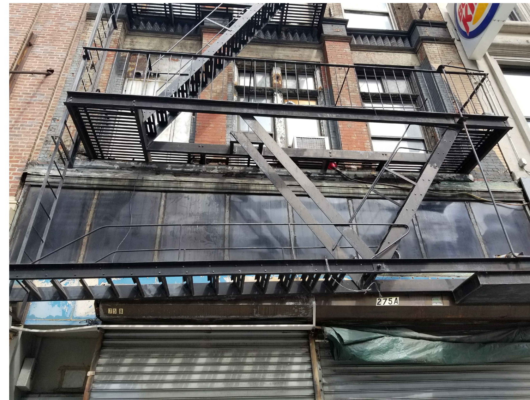
03 EXISTING CORNICE/SIGNBAND ABOVE STOREFRONT
